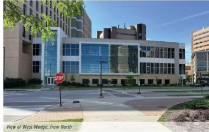
View of West Wedge, from North
