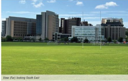
View (Far) looking South East
